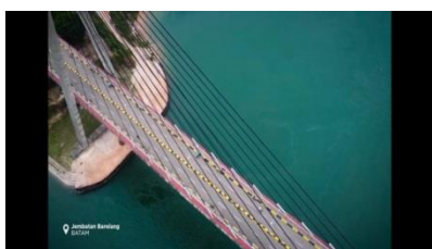
Frame 1. Belerang Bridge in Batam
